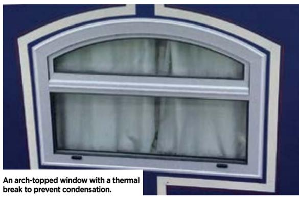
An arch-topped window with a thermal break to prevent condensation.
